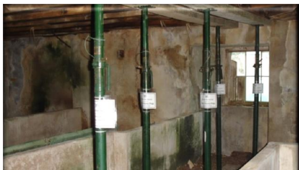
Sponsored Acrow props in place supporting the first floor.
